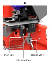
Fig 16.1 Filter dehydrator
