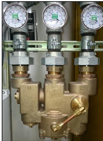
Figure 4. Blending Valve
