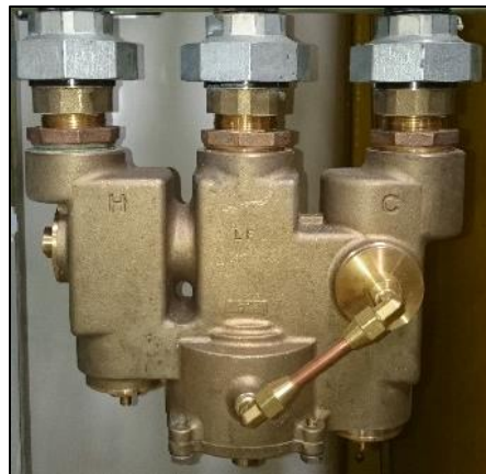
Figure 7. Blending Valve
