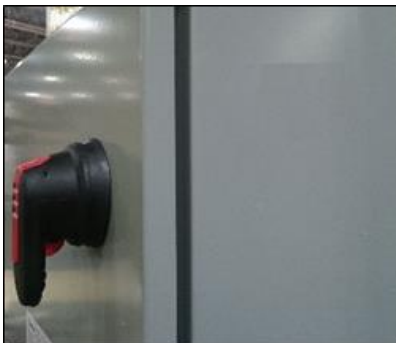
Figure 1. Disconnect Switch Junction Box
