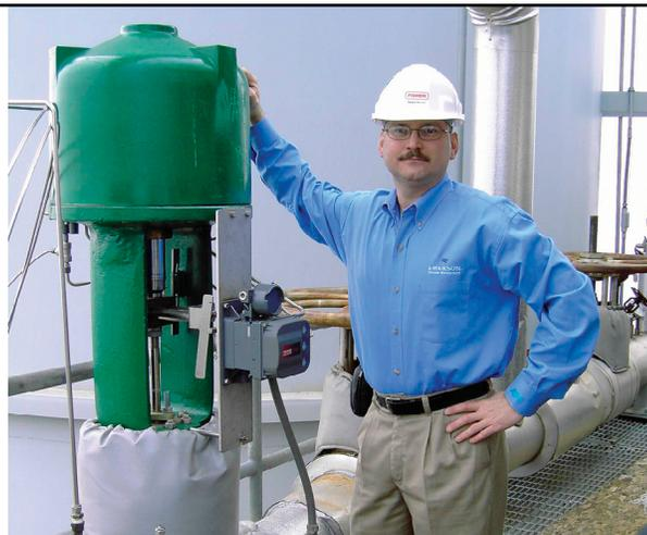
*Fisher™ HPT valves with Cavitrol™ III trim reduce cavitation and improve control in boiler feedwater application.*
